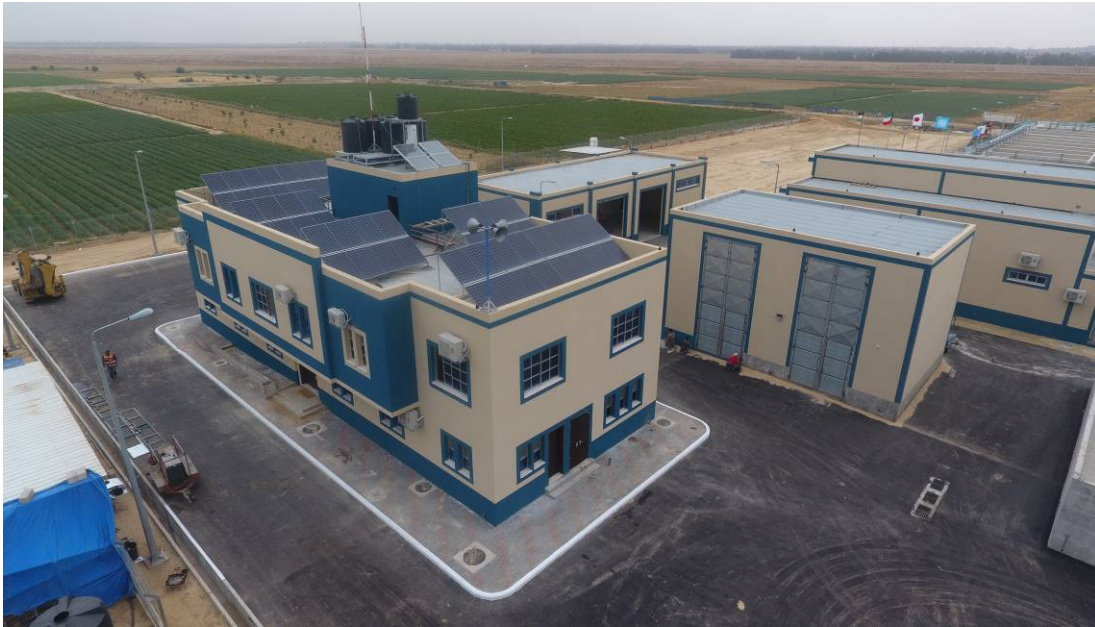
Accomplished Works of the Administrative Building up to August 2019
