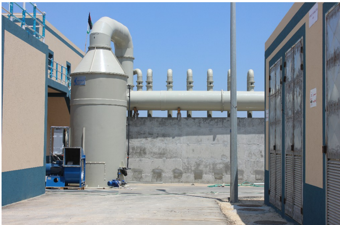
Structural and Mechanical Works for the Odour System up to August 2019
