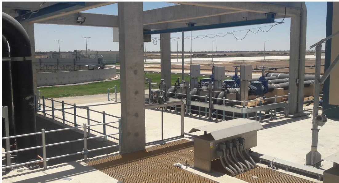
Structural and Mechanical Works for the Sand Filter up to August 2019
