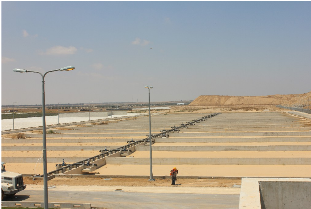
Accomplished Works for Drying Beds up to August 2019
