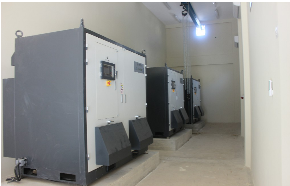
Mechanical and Electrical Works for the Air Blowers up to August 2019
