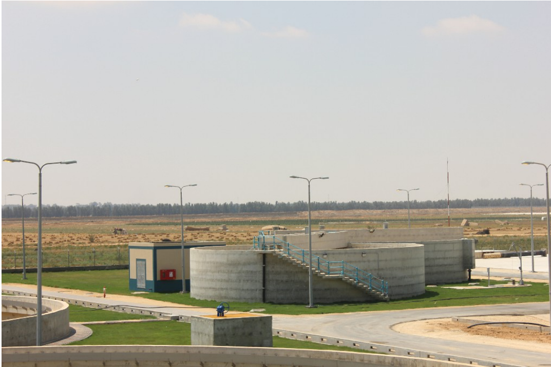
Structural and Mechanical Works for the Thickeners up to August 2019
