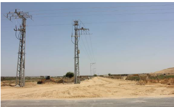
Installed Electrical Poles, Cables and Transformers of the Main Electrical Line up to July 2019
