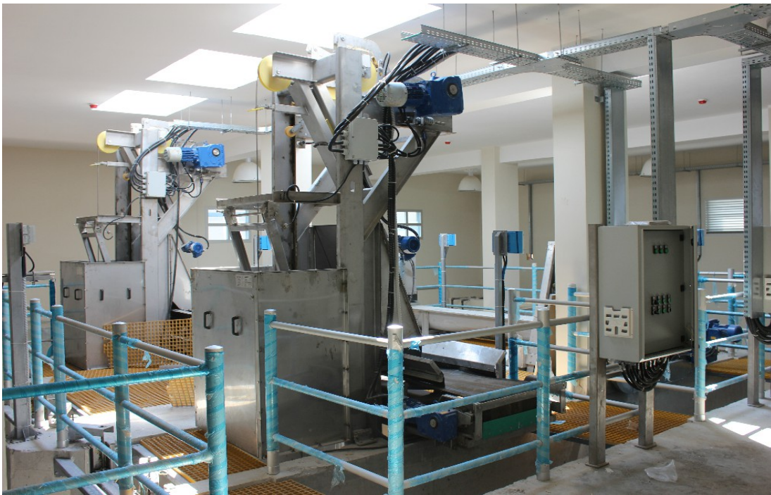
Structural and Mechanical Works for the Pre-Treatment Building up to August 2019
